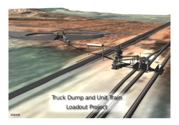
The project includes a new truck dump located on the east side of the highway, which would eliminate numerous daily at-grade highway crossings. Haul trucks would utilize the existing county road to just east of the highway where the trucks enter onto a new haul road that leads to a new truck dump and turn-around. Both products dump into a hopper from the haul trucks, screened, and then onto a belt conveyor that crosses over the highway to the new rail loadout facility.
